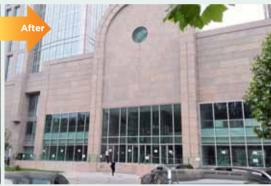
A portion of the rear stone wall was converted to glass curtain wall to create prominent frontage and visibility for the F&B units.
